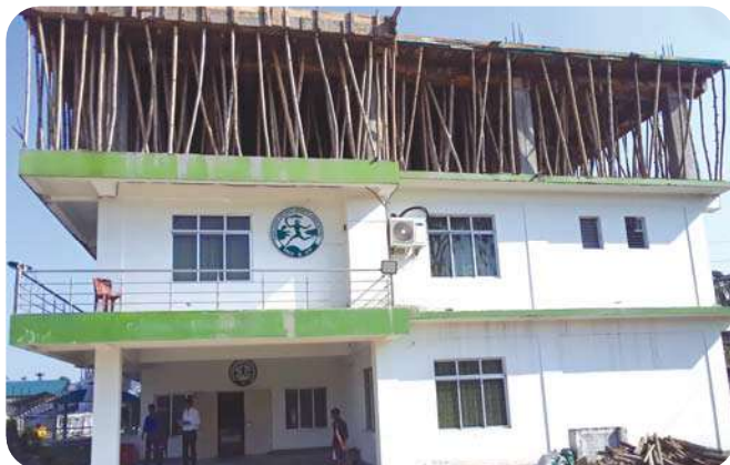
Infrastructure development of Jalan Nagar Outdoor Sports Complex at Dibrugarh
